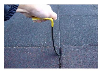
This will save the interlocks joints to be used again with the new (or same) unit being installed.
